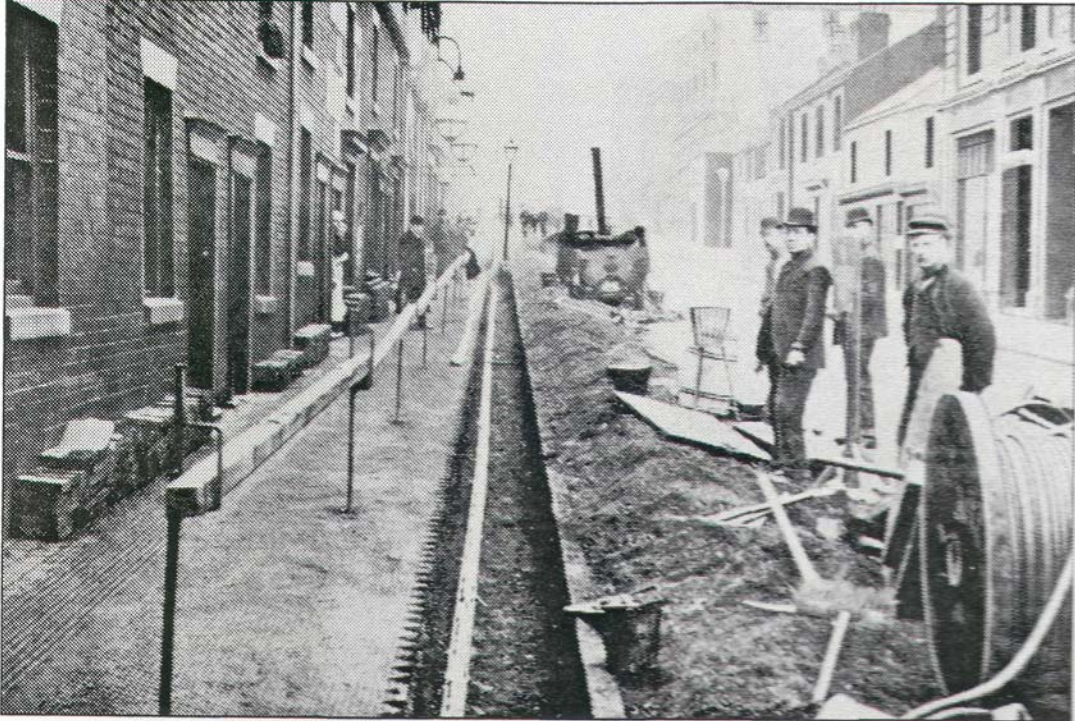
Cable laying at Hanley, Stoke-on-Trent, 1893
